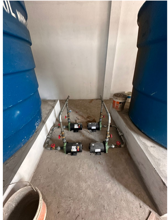
Fig. 38 – Bombas Cisterna
