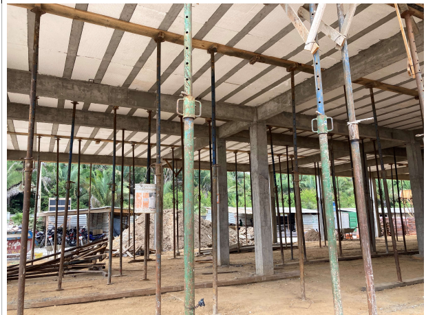
Fig. 2 – Laje concretada (SUGESQ)
